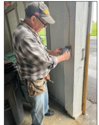
Paul Augsburger finishing up electrical installation work.
